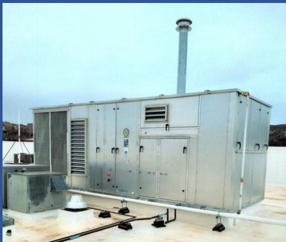
One (1) of four (4) large rooftop Air Handling Units (AHUs)
